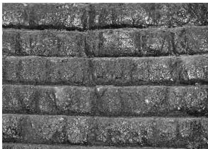
Figure 10. Photograph of the slag line lining (MC2) after 107 heats.
