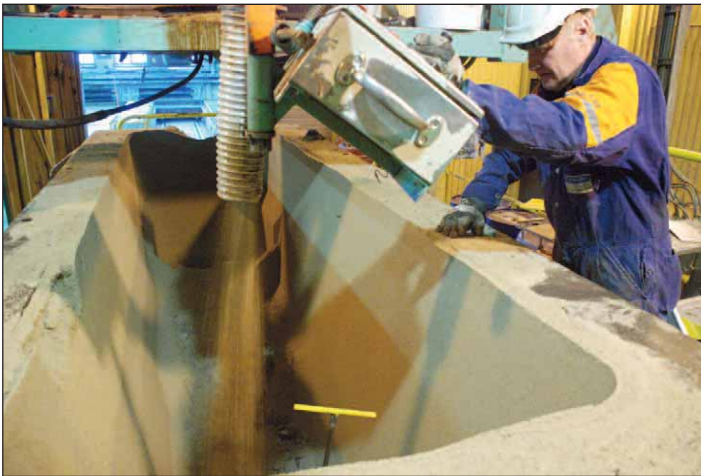
Figure 1. Installing a new EASYSET™ low VOC tundish working lining.
