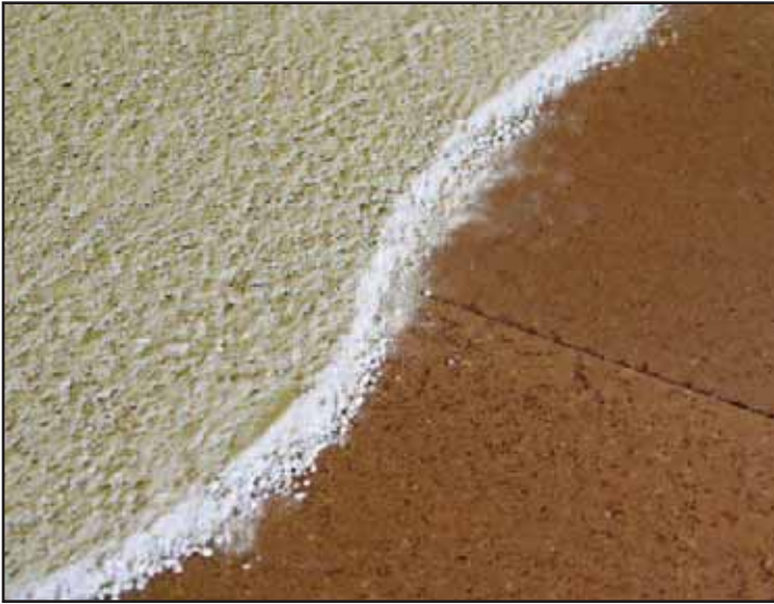
Figure 5. THERMTECH™ OLIBAR™ leveling compound over ALUBRICK™ cathode barrier bricks.
