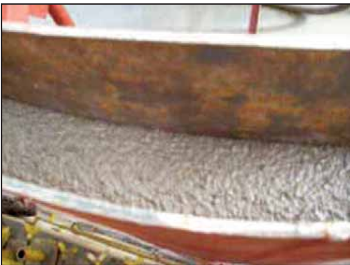
Figure 6. Gap completely filled up by castable.
