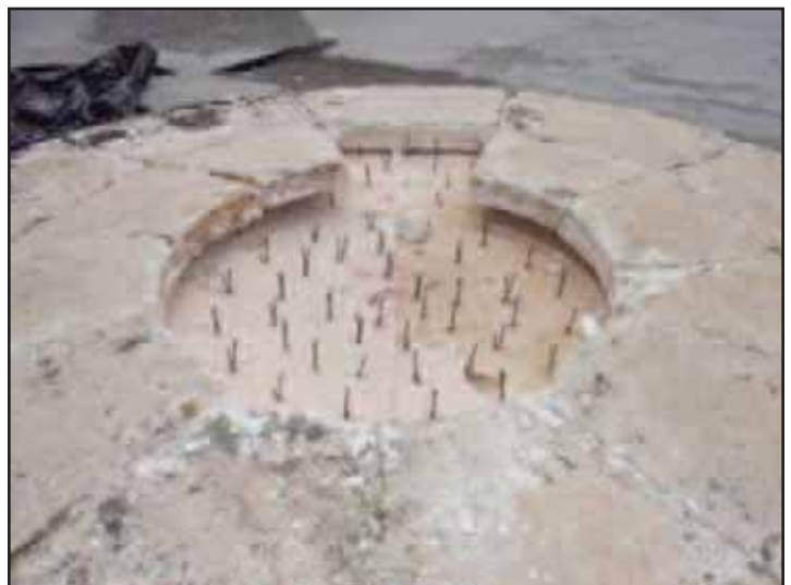
Figure 3. General view of damaged roof showing missing center panel.
