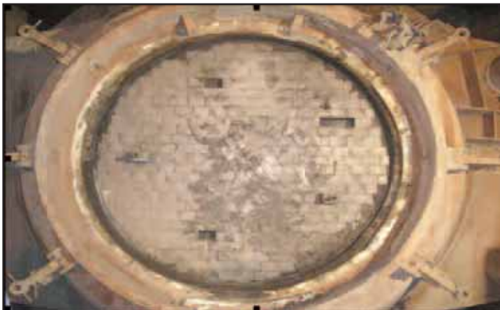
Figure 12. First inspection of the new R2U castable for removable bottom converter.
