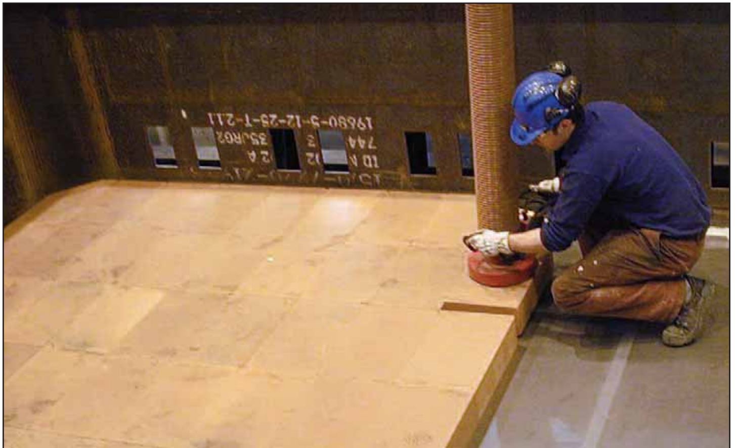
Figure 4. Relining an aluminum reduction cell with large format ALUBRICK™.
