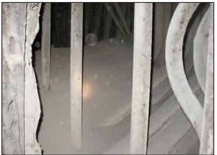
Figure 14. Typical upper frontwall dead air space (note fly ash).
