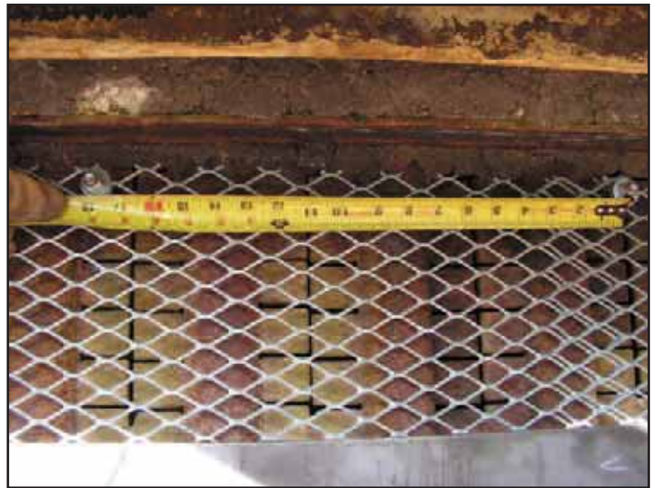
Figure 18. Nut and stud with washers holding expanded metal.
