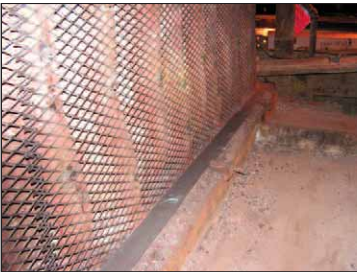
Figure 17. Expanded metal welded directly to tubes.
