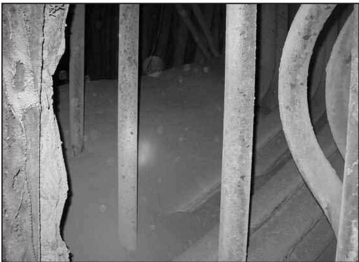
Figure 4. Typical upper frontwall dead air space (note fly ash).
