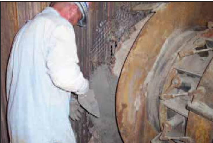
Figure 9. Typical pulverized coal type burner inside a windbox (note expanded metal welded to tubes around burner).
