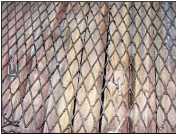
Figure 16. Insulation stud and clip used for holding expanded metal.
