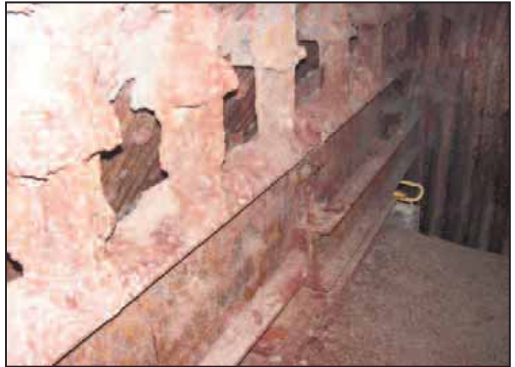
Figure 10. Typical structural supports inside a lower vestibule.
